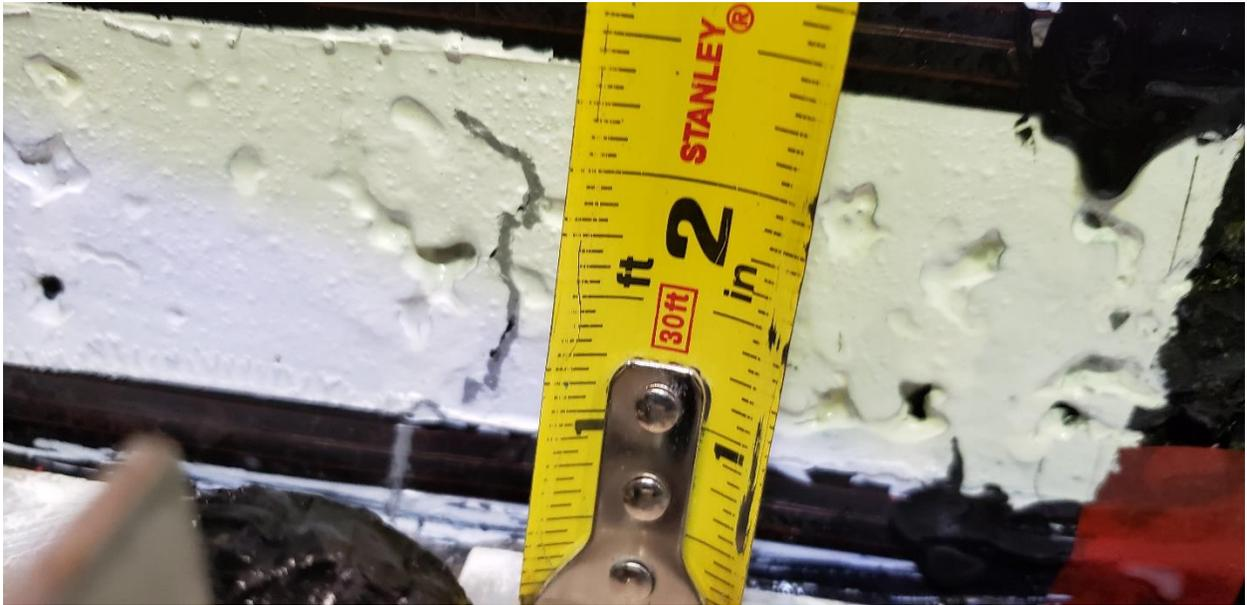
Fig 2 Bottom-up crack at SG6-N-0
