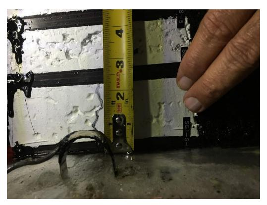
Fig 4 Bottom-up crack at SG1-S-0 2.5 inch long
