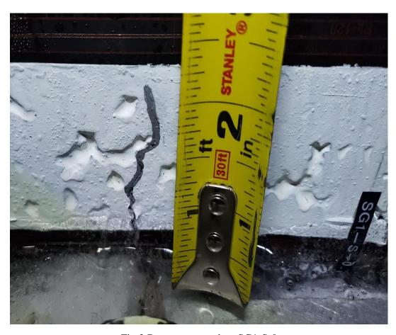
Fig 3 Bottom-up crack at SG1-S-0
