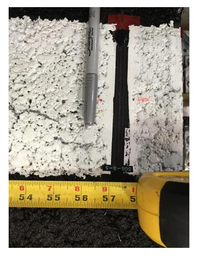
Fig 7 South section surface crack 3.5 inches from the outer vertical edge
