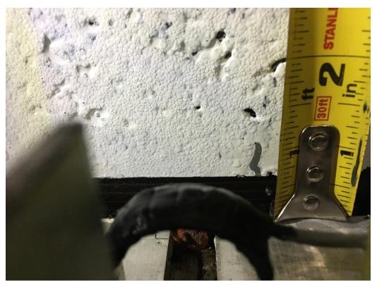
Fig 6 Bottom-up crack at SG6-S-0 1.0 inch long
